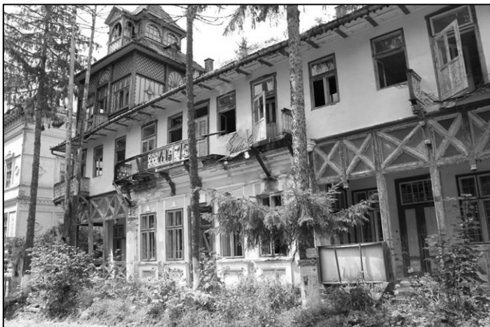
Figure 3. Historic villas in 7 Springs Alley in an advanced state of decay
