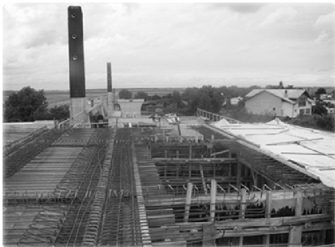
Figure 10. Bucharest-Braşov Highway Construction Works
