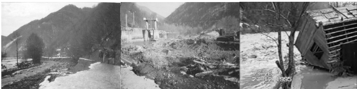
Figure 5. Problems created by the flood of December 1995, in the meadow of the Someșul Rece. 1. Damaged road near Măguri-Răcățău; 2. Clogged intake of Someșul Rece II; 3. House carried by flood.
