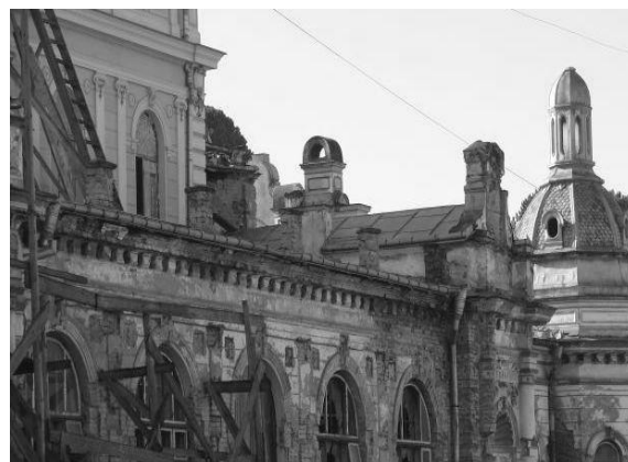
Figure 4. The Casino of Vatra Dornei at present
